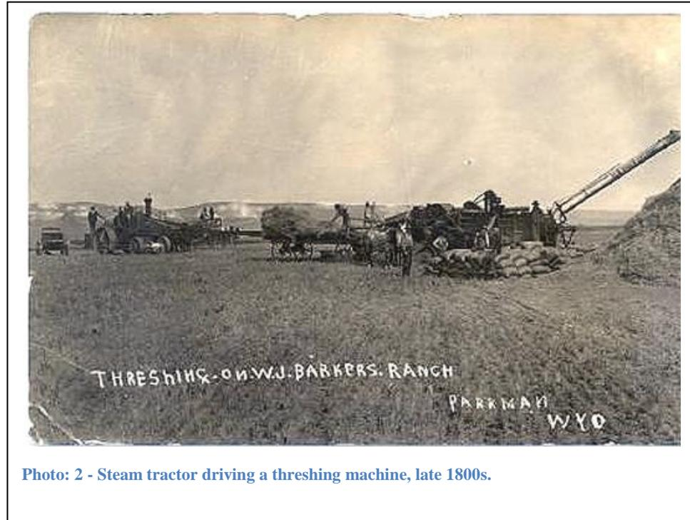
Photo: 2 - Steam tractor driving a threshing machine, late 1800s.
